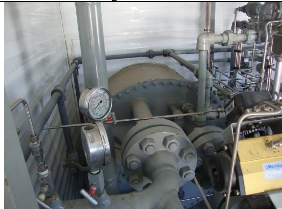
Vessel inlet piping
