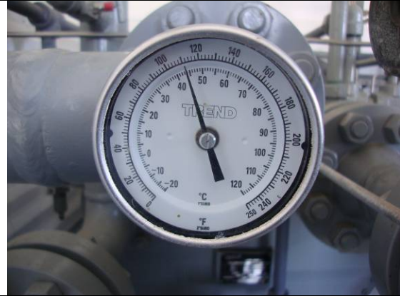
Vessel temperature gauge
