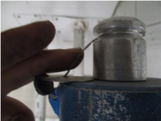
PSV SEAL WIRE INTACT
