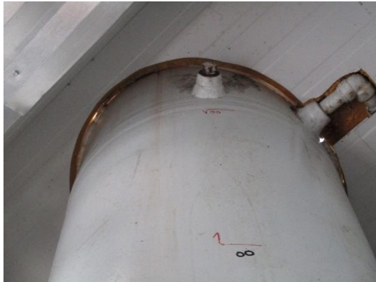
VESSEL THROUGH ROOF SEAL FAILURE
