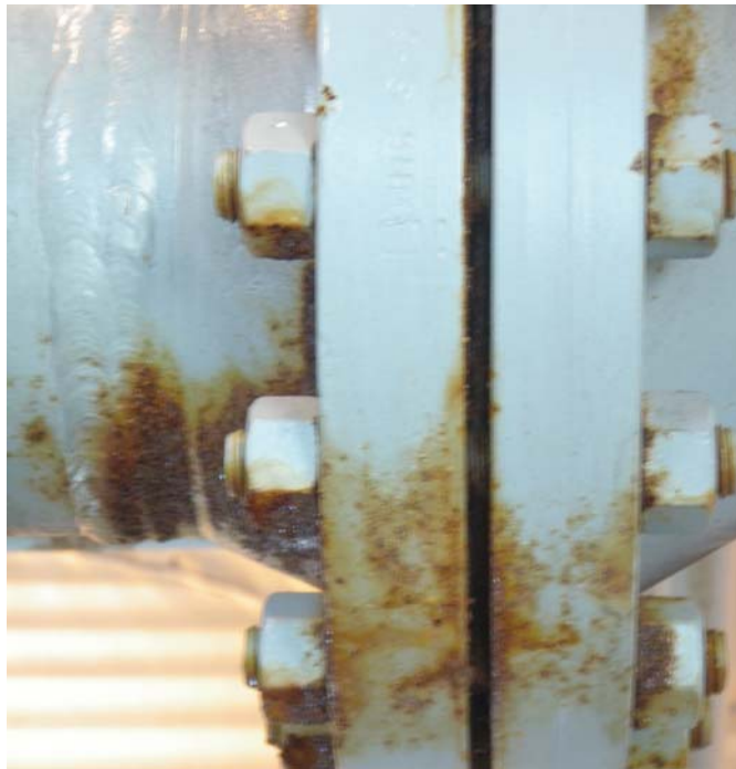
08-A0419464 Inlet Flange Surface Corrosion
