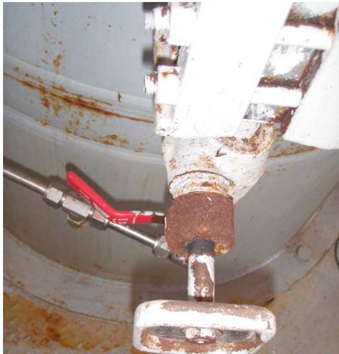
10-A0419464 Liquid Level Valve Packing Corrosion
